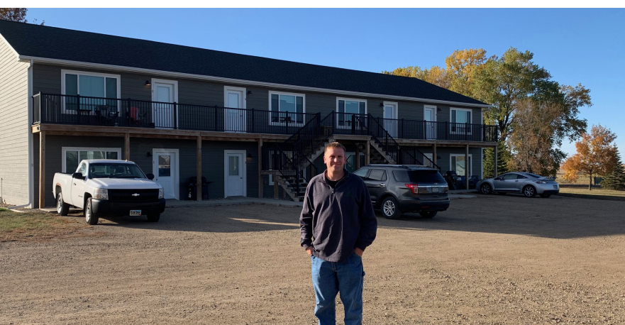
Jason Aho, mayor of Lake Norden, S.D., stands in front of a recently built housing development. Agropur's major expansion of the Lake Norden plant created the need for additional employees and spurred significant economic development in the city and surrounding region.
