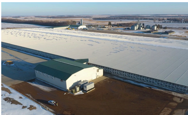
Garfield Dairy, located outside Bryant, S.D., will provide its milk to Agropur's Lake Norden plant. It's the largest, single-site dairy farm in South Dakota.
